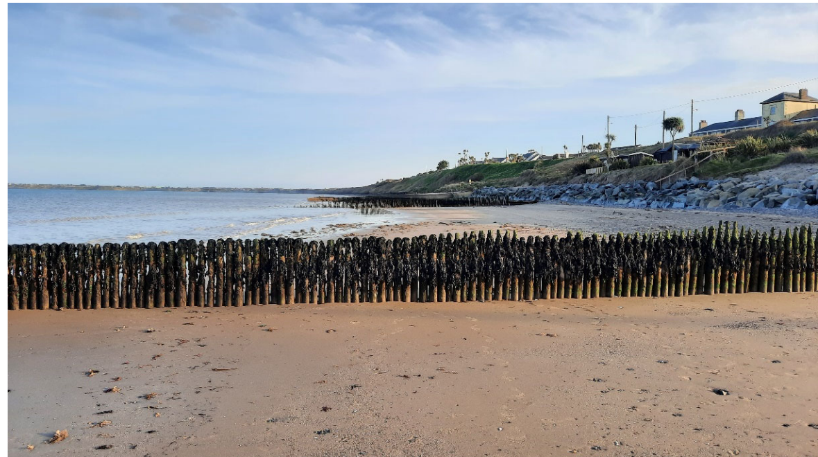
Remnants of 1950s timber groynes
